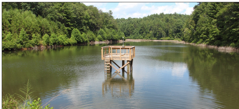
Burson Pond. All that's left of the covered pier.
