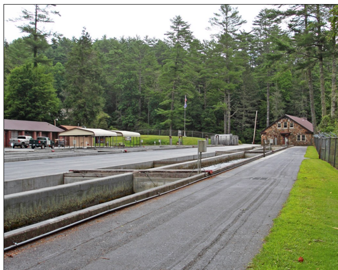
These long concrete pools of cool running water contain millions of trout in various stages of development. The fish are very spooky so they ask that you do not harass them. There are no barriers so you do need to be very careful with children.
